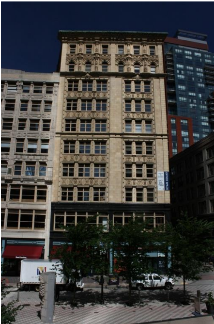
Figure 3. Washington Street (east) façade.
