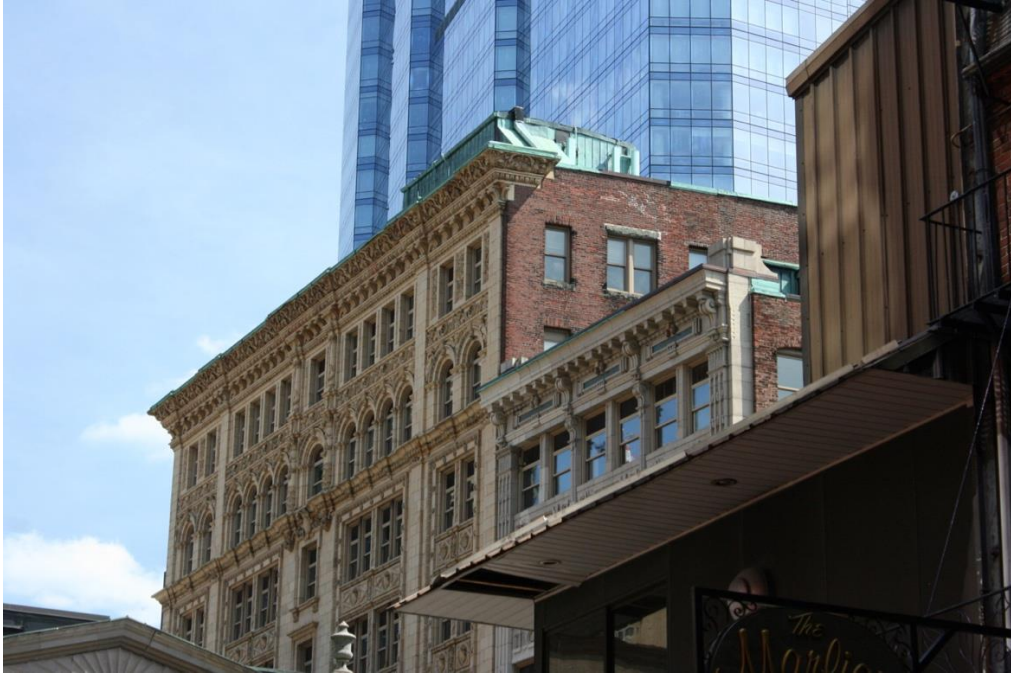
Figure 10. Bromfield Street (north) and west elevations.
