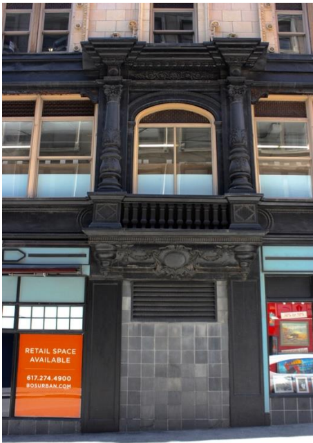
Figure 11. Bromfield Street building entrance.
