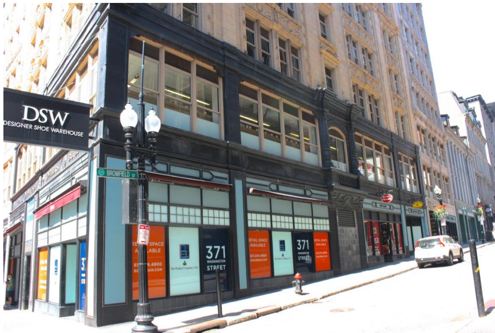
Figure 5. Bromfield Street facade, storefronts.
