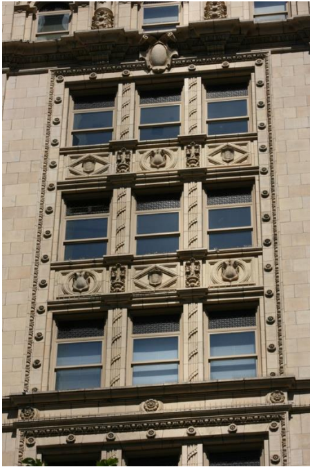
Figure 7. Washington Street façade, detail of floors 6, 7, and 8.
